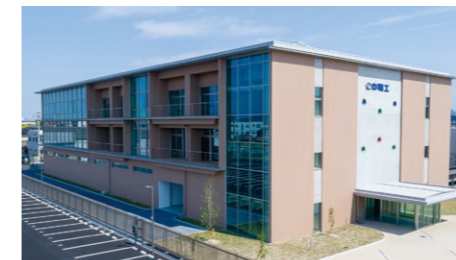
Okayama Supervising Branch Completed: April 2019 Standard: ZEB Ready Total floor area: 4,836m 2 (3 stories)
