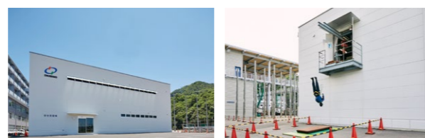
Practical Safety Training Building
