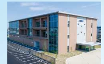
Constructed a new ZEB-compliant building for the Okayama Supervising Branch (2019)
