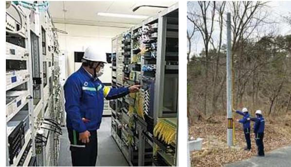
An inspection in progress
