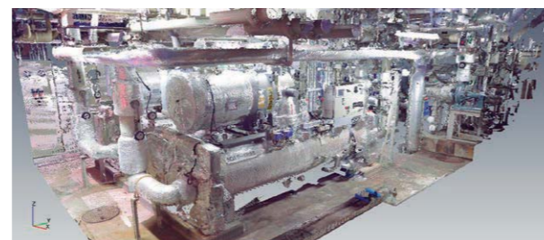
[3D点群データ] 3次元位置情報をもった点に着色したもの。 [3D point clouds] An image acquired from colored points with 3D position information.
