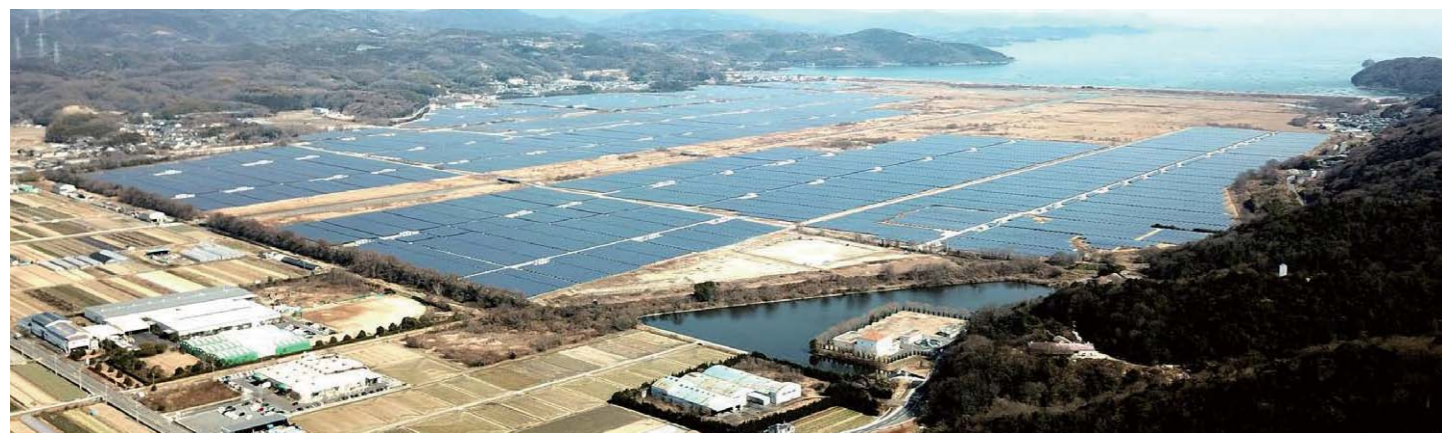
瀬戸内Kirei太陽光発電所(岡山県) Setouchi Kirei Mega Solar Power Plant (Okayama Prefecture)
