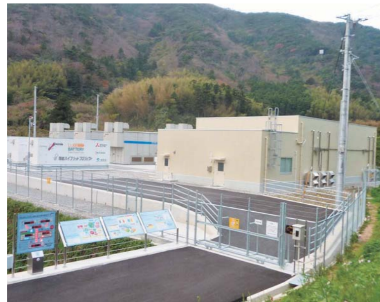
西ノ島変電所(ハイブリッド蓄電池システム)新設工事(連携設備)(島根県隠岐郡) New construction (coordination facility) at Nishinoshima Substation (Hybrid Battery Storage System) (Oki District, Shimane Prefecture)
