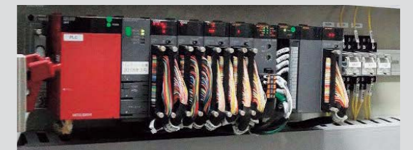
■ PLC(盤内) PLC (inside the panel)
