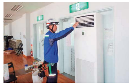
避難所へのエアコン設置工事 Air conditioning installation at evacuation shelter
